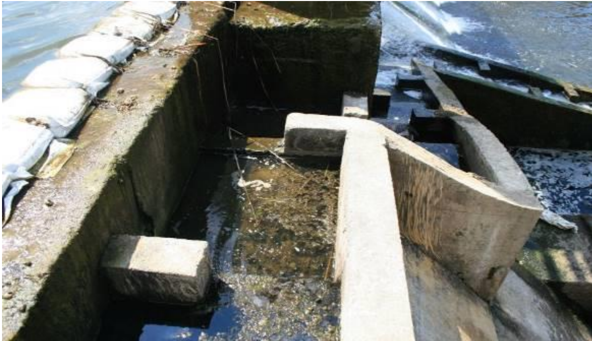
Fish passage, Nikolaevo fishponds weir, Tundzha River at Zhrebchevo SPA
