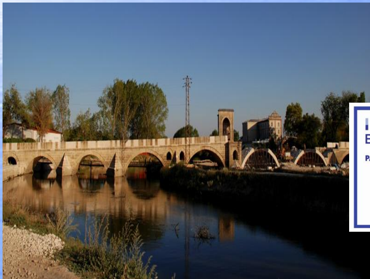
A photo of TUNCA BRIDGE during restoration
