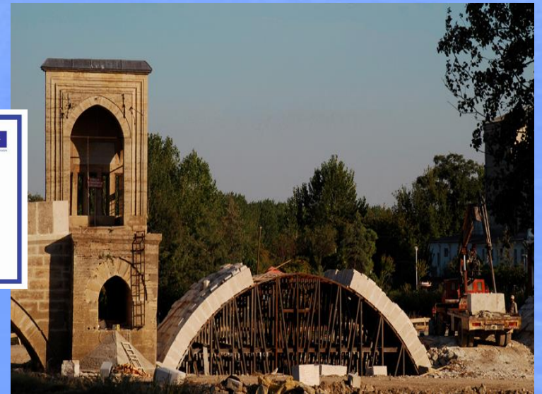
A photo of TUNCA BRIDGE during restoration
