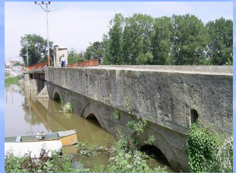
A photo of TUNCA BRIDGE before restoration
