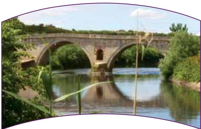
Мостът Акарджа - ( http://www.tgdturkey.com/tr/kirklareli/foto-galeri/pehlivankoy-akarca-koprusu/pehlivankoy-akarca-koprusu-1.html )
